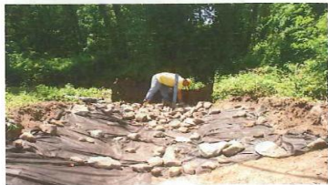
What does hand placing the rip rap mean?. Photo courtesy Pat Rector May 2011
