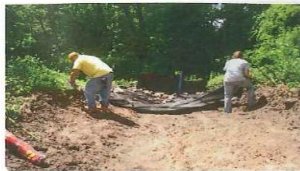
Chris and Jillian Thompson putting up silt fence. Photo by Pat Rector May 2011.
