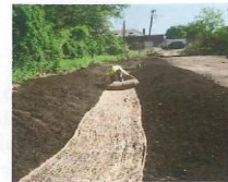
Laying jute Photo by Pat Rector May 2011.
