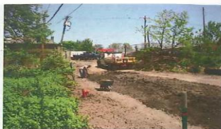
Adding soil for the berm. Photo by Pat Rector May 2011.
